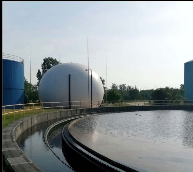
Urban Wastewater Biogas Plant
